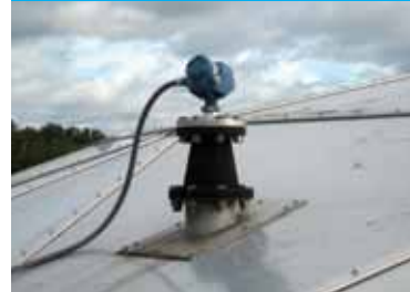
5400 Sludge holding tank
