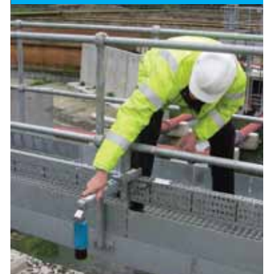
3107 Pumping station level
